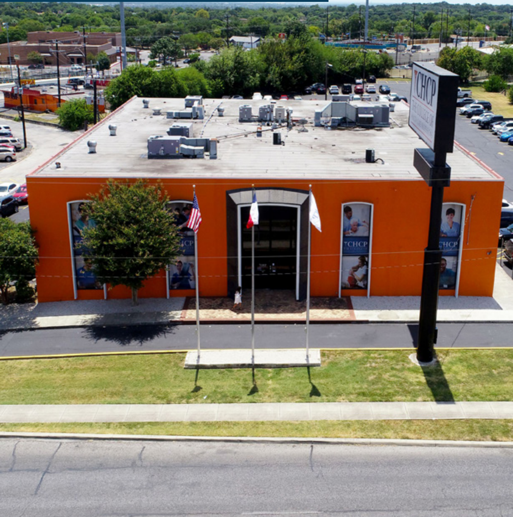
HIGH VISIBILITY OFFICE | 4738 NW Loop 410, San Antonio, Texas
